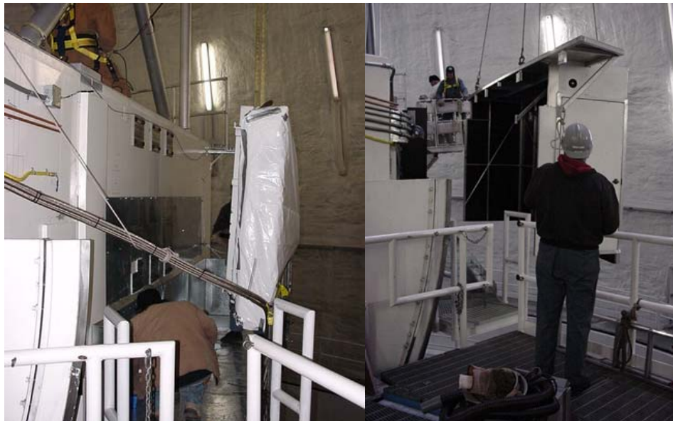
Figure 6: Laser Mounting onto Elevation Ring
