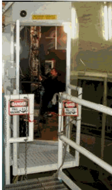
Figure 5: Laser Service Enclosure and Optical Bench for the Keck II Laser System
