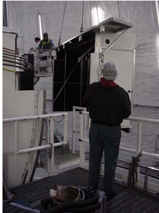
Figure 3: Laser Enclosure Structure
