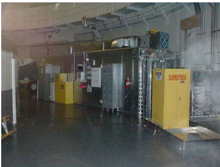
Figure 5: Laser Room on Dome Floor
