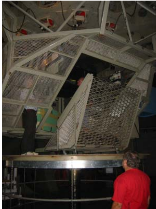
Figure 14: Installation of the Cassegrain cage door
